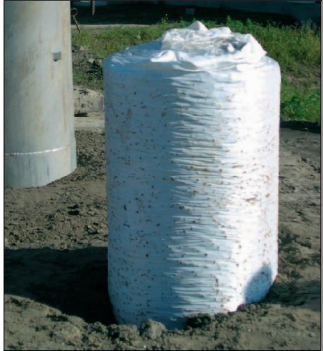
Figure 6. Installed GEC at Bastion East
